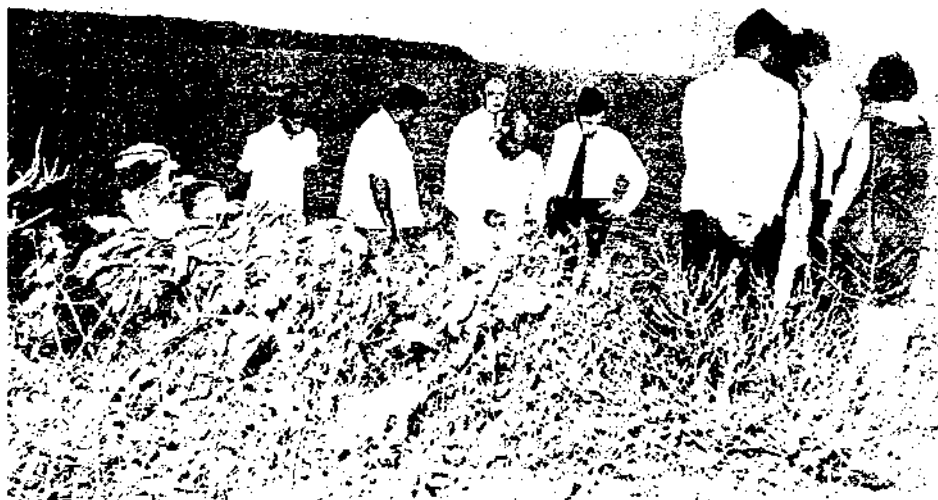
Visitors at the proposed site for the NIO buildings, Panaji, Goa.
