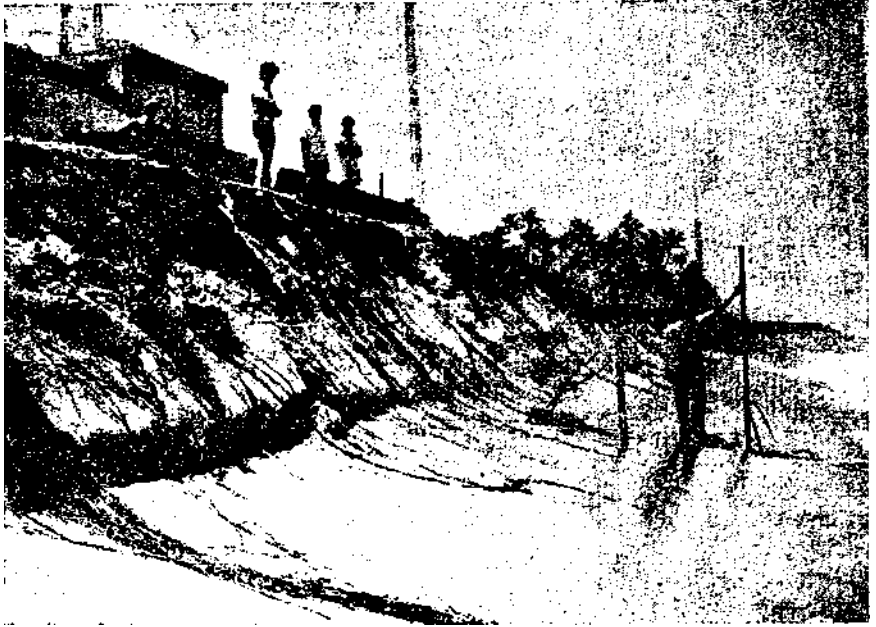
Severe erosion of the Thumba Beach (Trivandrum).
